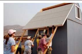
Final Roof Section
